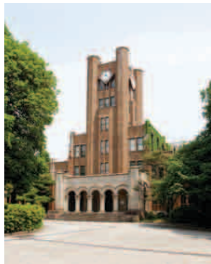
Building 1 of the Komaba Campus is used for lectures. The clock tower has become the symbol of the campus.
