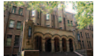
III / GSII Main Building.
