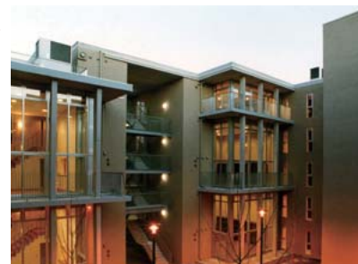
Toshima International Hall of Residence
