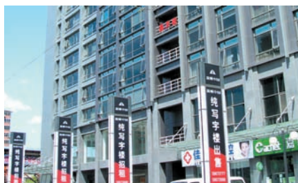
Beijing Office is located in the building 'Freetown' in southeastern Beijing
