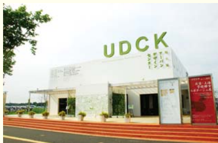
External view of Urban Design Center Kashiwanoha
