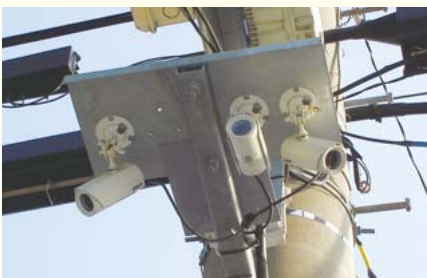
Security cameras on telephone poles around Kashiwanoha Station
