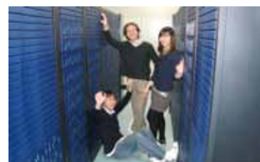
In the supercomputer room.
