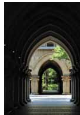
Arcade sidewalk at Faculty of Letters Bldg 2.
