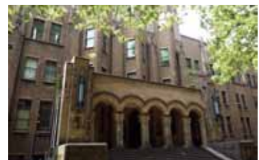
III / GSII Main Building.
