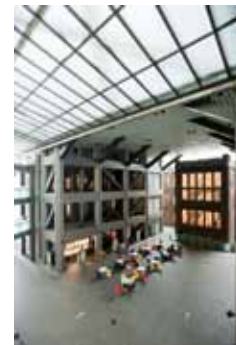
A blend of old and new, Engineering building No.2. The newer wing was built in 2005 to hover over the old wing, which was built in 1924.
