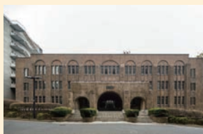
Faculty of Engineering Building 4
