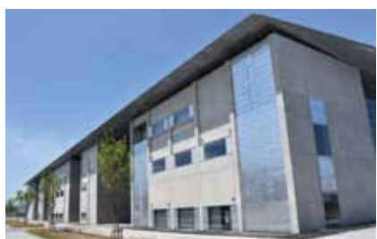
Research and Testing Complex I, IIS Chiba Experiment Station
