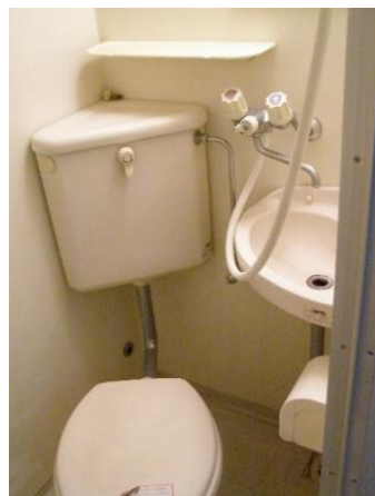
Fixed Type Bathroom (Building A & B)
