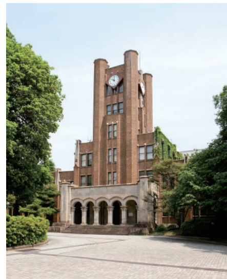
Building 1 of the Komaba Campus is used for lectures. The clock tower has become the symbol of the campus.
